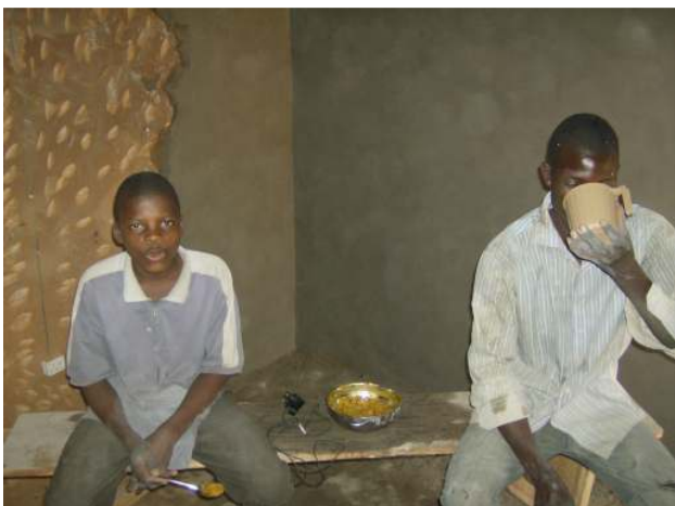
Plastering the inside of the building
