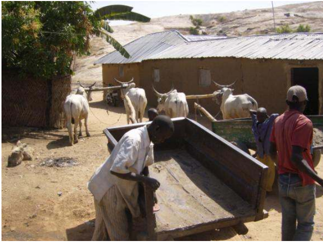
Delivery of sand to make cement to plaster the mud building to protect it from rain in wet season
