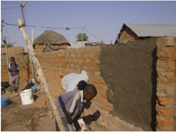
Plastering the compound wall
