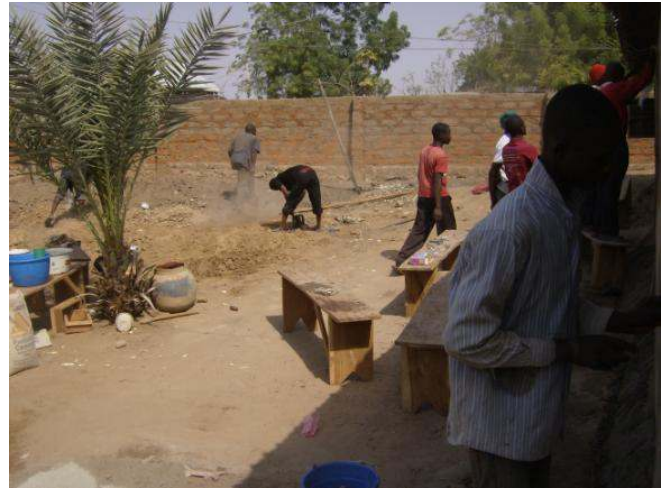
Renovating the yard
