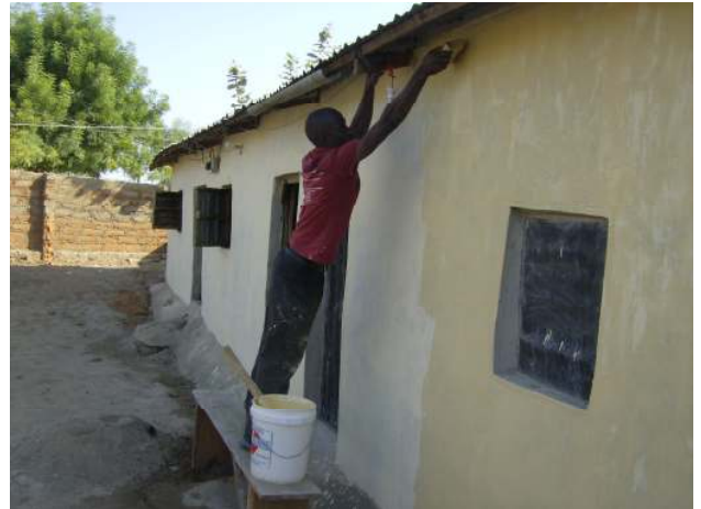
Plastering, then painting the outside building
